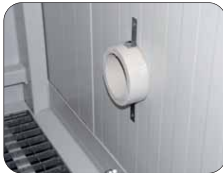
K-90 shut-off device
