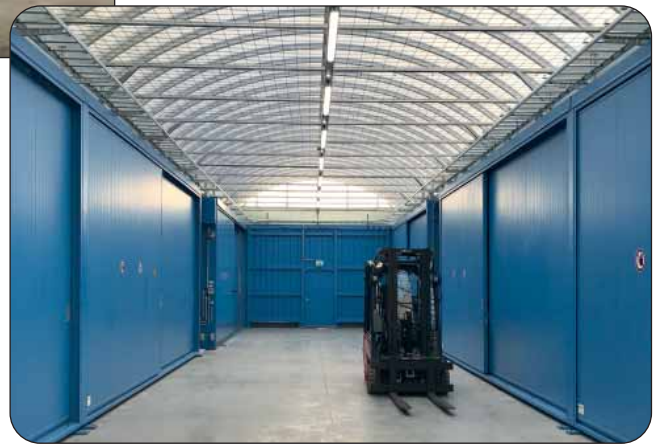
◆ Corridor closure ahead with sky light panel ◆ Corridor lighting
